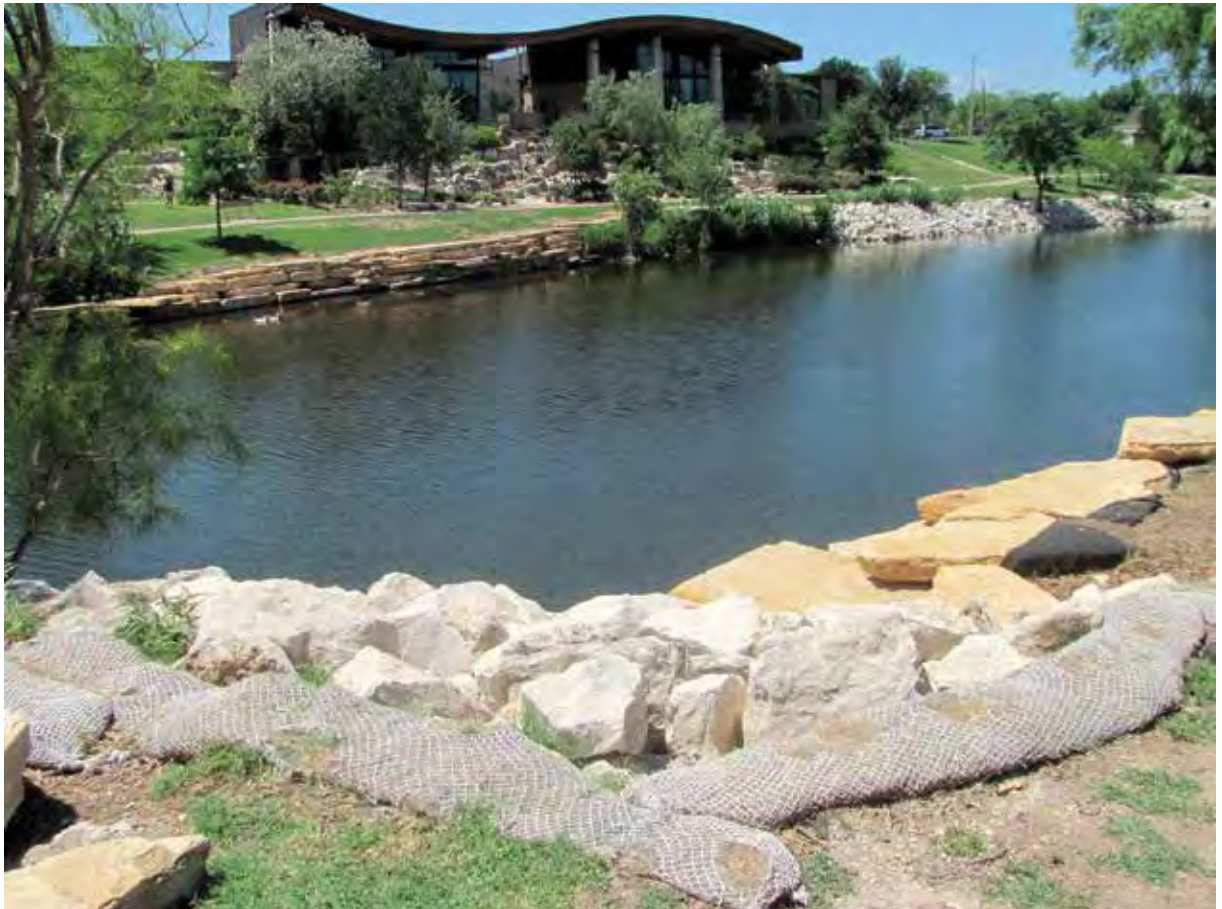
North Concho River with bank stabilizing BMPs (Source: UCRA)
